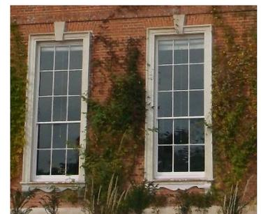
Stonework damaged through weathering and neglect has been sensitively repaired. The finished windows, right, show repairs to seals and dressings blend.
