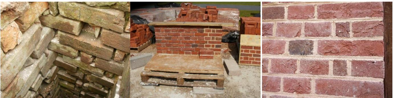
From left: The poor state of repair of brickwork. Commissioned bricks designed to match Renaissance originals in texture and colour. In situ in the new Loggia
