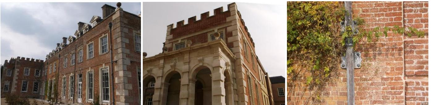
From left: The restored South Façade. The new build loggia and apartment. Seamless repairs and coloured pointing work on the weathered South Wing
