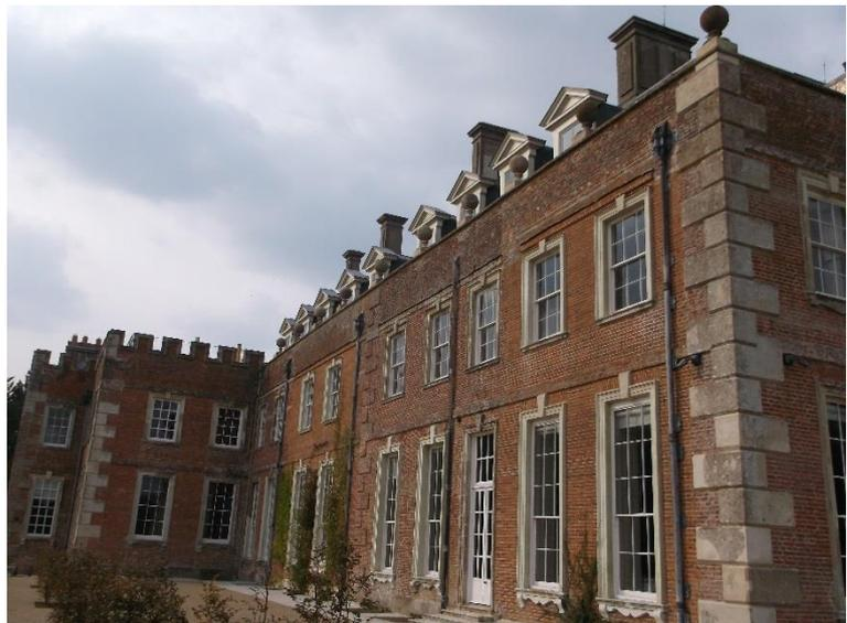
From left: The new loggia replicates the north door and stone is married in with specially commissioned brickwork. The South façade demonstrates replacements, and repairs to edging stonework, window seals, window dressings, and ornamental features on the roof.
