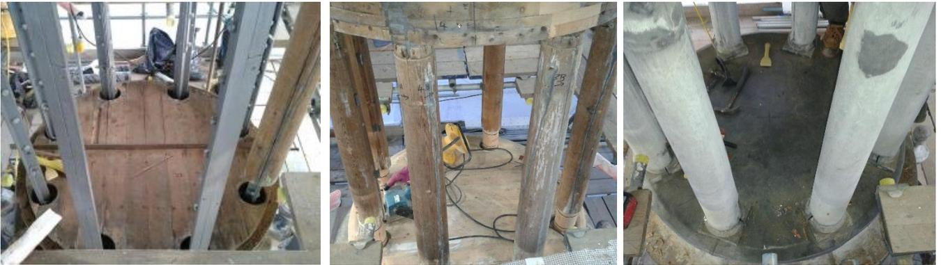
A new steel frame was commissioned to replace the perished ironwork Belvedere structure. This was craned into position, clad in timber, using original restored timbers where possible alongside new inserts, and then covered in lead in accordance with the original design.
