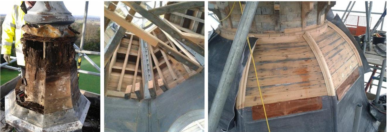
Lead and wood was eroded throughout the structure. What could be preserved was, and reclaimed wood was used alongside new materials to recreate the Belvedere wood clad and lead coated structure.
