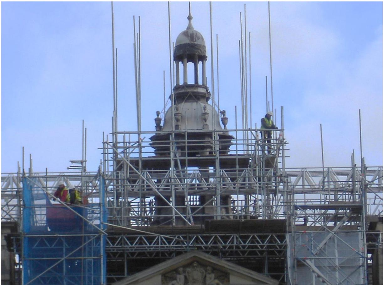
The original Belvedere Tower. The whole structure was removed, repaired and rebuilt and craned back into position.
