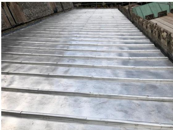
roof deck in the same way they would be on a traditional lead covered roof. The TCSS roll coverings are manufactured to give watertight seal between the bays. The bays for the Pewsey project were measured on site and manufactured in our workshop in Shepton Mallet. Due to the considerable weight saving, these could be transported using a van.
