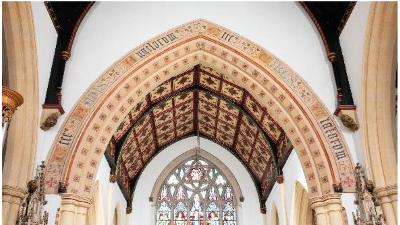
The original ceiling was reinstated and its timber surfaces were repaired and re-varnished. The church floor was relaid. Old red carpeting was removed and the parquet floor repaired. New carpet was laid and tiles to the sanctuary and re-finished floor boards to the Sacristy were finished with oak detailing and trim.
