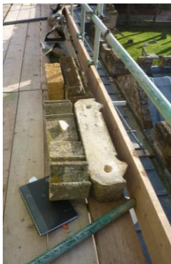
Masonry repairs in progress left and middle, and right after repair.
