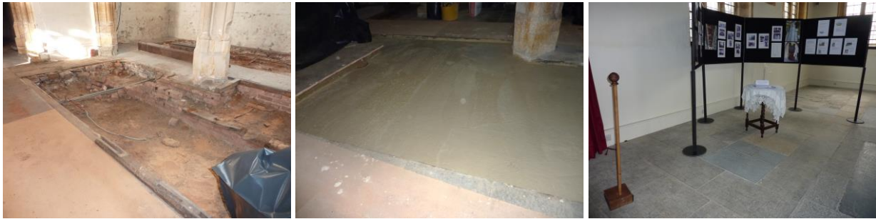
Before, during and after floor repairs.
