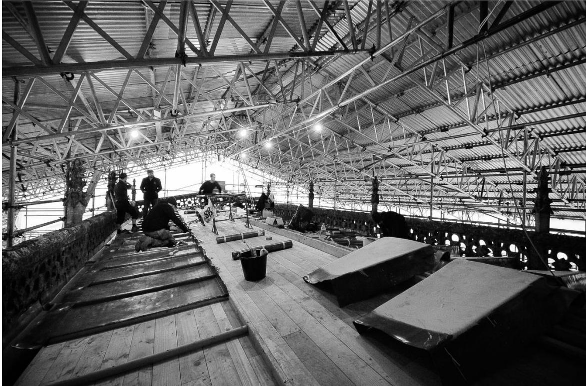
St Marys Church, Batcombe is a Grade I listed church in Somerset dating to the 15<sup>th</sup> and 16<sup>th</sup> centuries. It is built of rubble, ashlar and dressed with local Doulling stone. In 2017 we re-laid the Nave and Aisle lead roofs and repaired masonry. We erected a temporary roof to protect the Nave, and Aisle roofs, then lifted and replaced the eroded lead.
