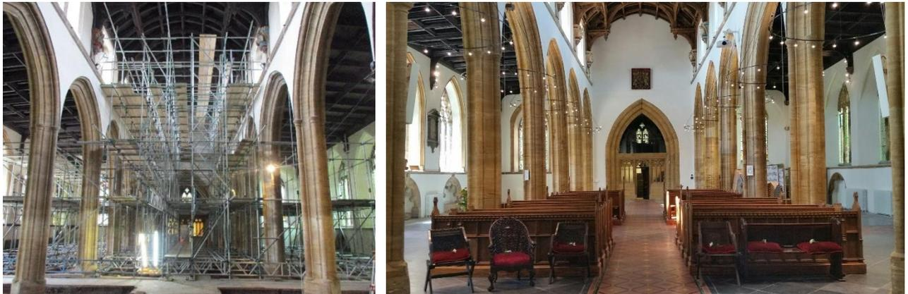
St Mary's Church is Grade I listed building dating from the 13<sup>th</sup> C with a Victorian styled interior. Ellis and Company were principle contractor to reorder the church for contemporary use by completing a programme of structural repairs and underpinning, laying a new stone floor, installing heating, lighting sound and catering facilities, and conservation cleaning historic timber ceilings, fittings and lime rendered walls.
