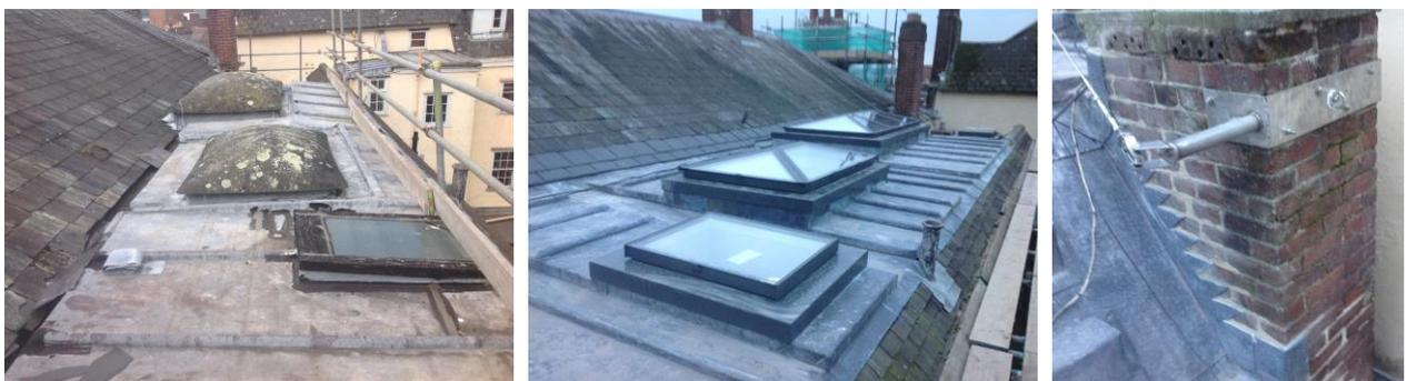
Left and Middle: Before and after two rows of slates replaced, new rooflights and releading. Right: chimneys were repaired and structural steel supports were installed for safety of future access.
