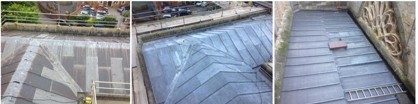
Left and Middle: Pitched roof before and after. Right: a further area of lightly pitched roof after releasing.
