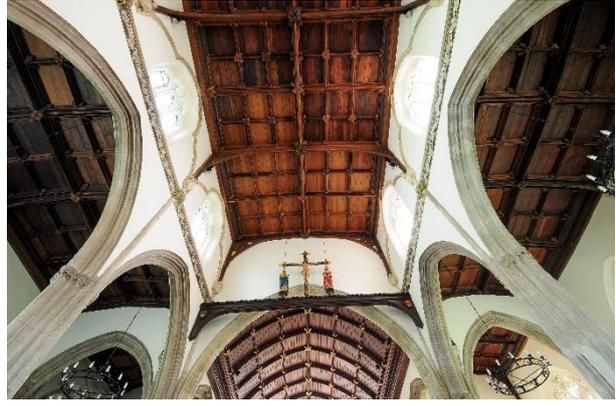
Layers of dark waxy dirt meticulously removed from the timber ceiling using a combination of conservation methods. The church was redecorated throughout including the repair and gilding of decorative details in the timber ceiling.
