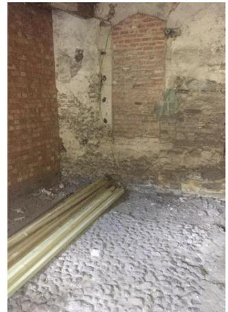
The ground level was excavated and drainage installed. The floors were then relaid with a deep mineral wool insulation and wooden floor boards, vinyl floor coverings were laid in the bathrooms. And the original flint floor was retained in the entrance and repointed with lime and grit mortar.
