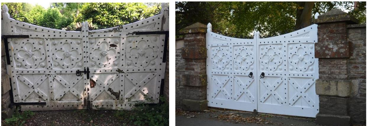
*Before (left) the old rotted gates as shown above and after (right) after restoration.*
