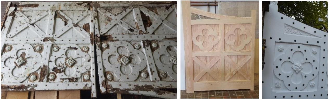
*Before (left) the rotted gates. (middle) the newly constructed gate structure (Right) with the addition of recovered decorative details and studs, repainted and rehung.*
