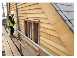
The chimneys were partially rebuilt down to the roof line and refitted with flues. During structural repairs to the walls it was discovered that a supposed brick wall was an original timber framed construction. The wall design was adjusted to be timber-lined rather than lime rendered in keeping with the original construction.
