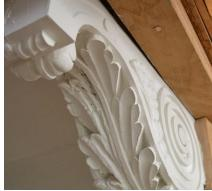
In addition to roofing, slating, leadwork and masonry the repairs timber repairs included removing paint from the corbels to reveal the decorative carvings underneath and replacing damage elements with newly carved inserts.
