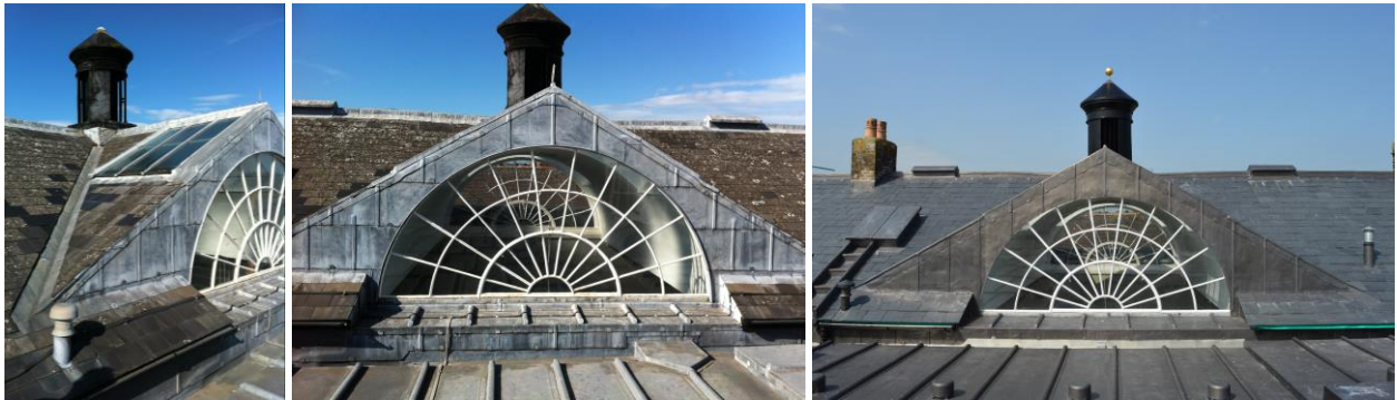
Before and after slating, leadwork and glazing repairs
