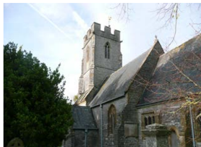
Before work commenced
