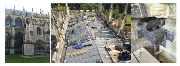
We carefully removed the existing flat roof structure and associated steel and brick work above the St Andrew and St Catherine chapel while retaining and protecting the chapel ceiling.
