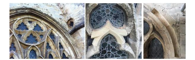
The medieval clerestory window was also subject of a conservation research project. After the stained glass had been cleaned and conserved, a single supplementary light of protective glazing was installed in a trial area to establish the effectiveness of its protection from condensation, and the aesthetics of different glazing treatments using horticultural glass sheet, bronze t-bars and leaded samples following the line of the medieval lead.
