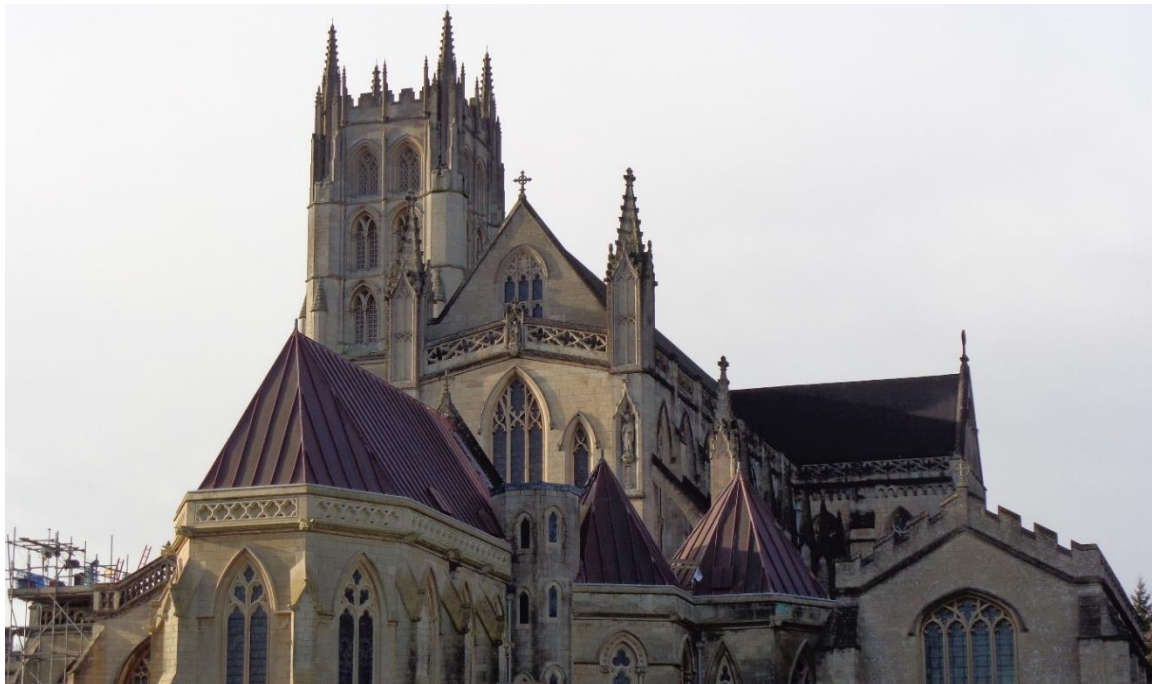
Downside Abbey Restored
