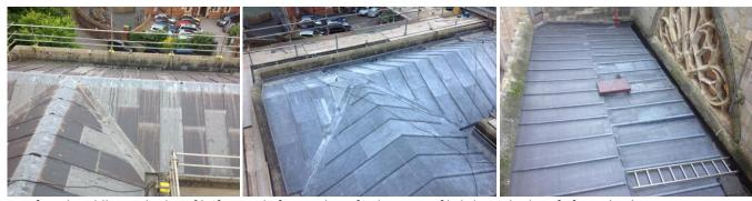
Left and Middle: Pitched roof before and after. Right: a further area of lightly pitched roof after releading.
