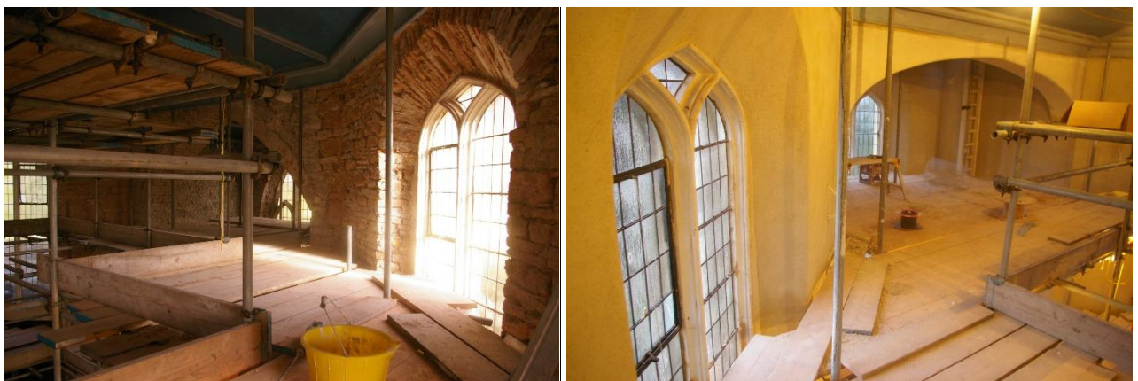
Internal masonry was repaired, lime plastered and painted in conservation paints
