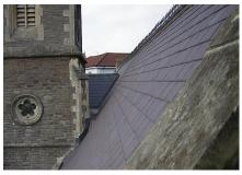
Slate roof tiles were removed, assessed, repaired where possible, and replaced alongside modern additions. New Welsh Penryn Blue Slates were chosen to blend with existing tiles in colour, size and texture. An alternative and cost effective Spanish Slate was used in less visible areas. Decorative ridge tiles which once adorned the roof crest were recovered, repaired and replaced thus restoring a classical Victorian feature.
