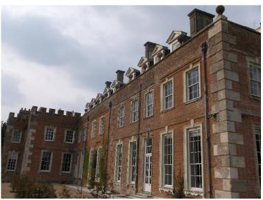
From left: The new loggia replicates the north door and stone is married in with specially commissioned brickwork. The South façade demonstrates replacements, and repairs to edging stonework, window seals, window dressings, and ornamental features on the roof.
