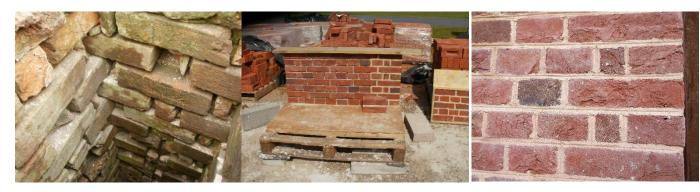
From left: The poor state of repair of brickwork. Commissioned bricks designed to match Renaissance originals in texture and colour. In situ in the new Loggia
