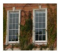
Stonework damaged through weathering and neglect has been sensitively repaired. The finished windows, right, show repairs to seals and dressing blend.
