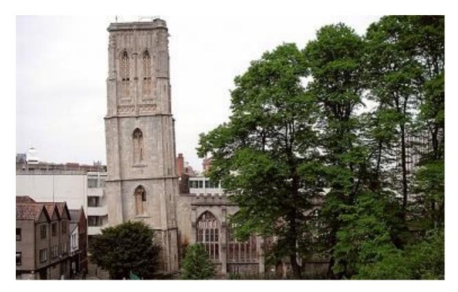
English Heritage and Architects Philip Hughes Associates contracted Ellis and Co to repair masonry on each elevation. We worked around the tower two elevations at a time cleaning and repointing the stones. Loose stones were fixed and missing stones carved and replaced by our masons. Structural pins were inserted where required. New panels moulding were carved for the belfry windows. Structural roof timbers were repaired by our joiners and a new lead roof was fitted.
