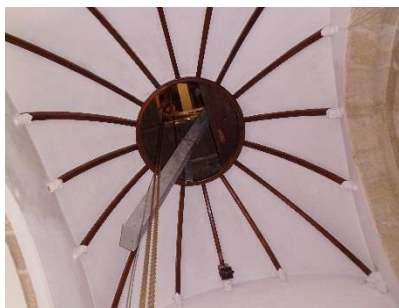
Steel beam being raised through the bell tower. The new steel and timber construction will hold the bell tower together.
